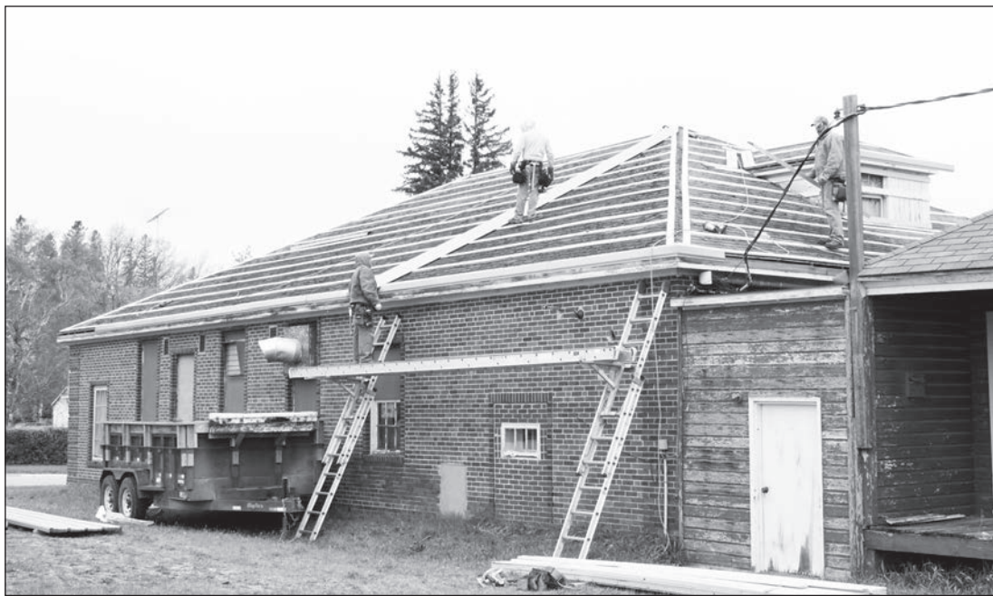
Friborg Contracting of Bagley was hard at work Friday, May 8 th replacing the old, shingled roof with new steel on the old creamery building. The Gonvick Co-op Creamery was sold to Land O'Lakes Creameries, Inc. in February 1971. In the late 1970's, the Gonvick-Trail School District purchased the creamery building and remodeled it into a vocational center for high school students. Now it is privately owned.
