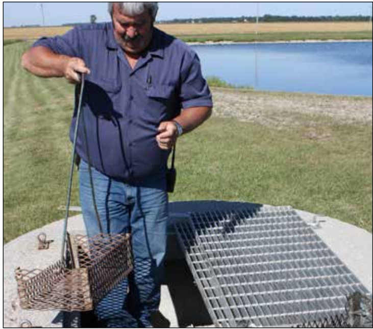
New screen ready to be lowered to catch the wipes and debris coming out of the sewer pipe into the ponds.
