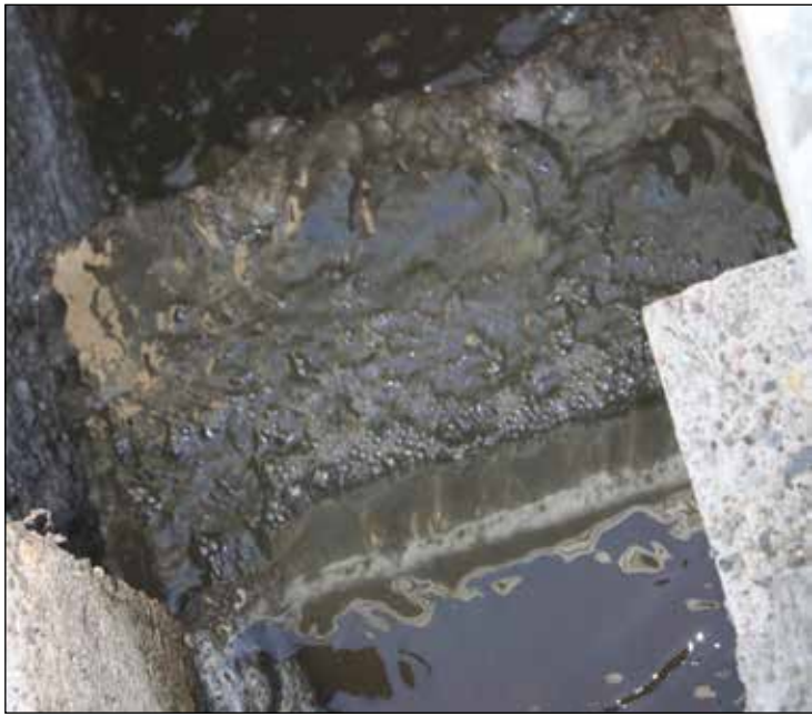
Water coming into the Oklee ponds must go through a screen to catch all the wipes and other things that should not be flushed.
