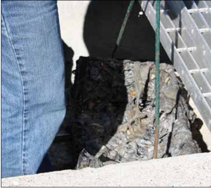
The screen being pulled out to be replaced with a cleaned screen. This is done twice a week.
