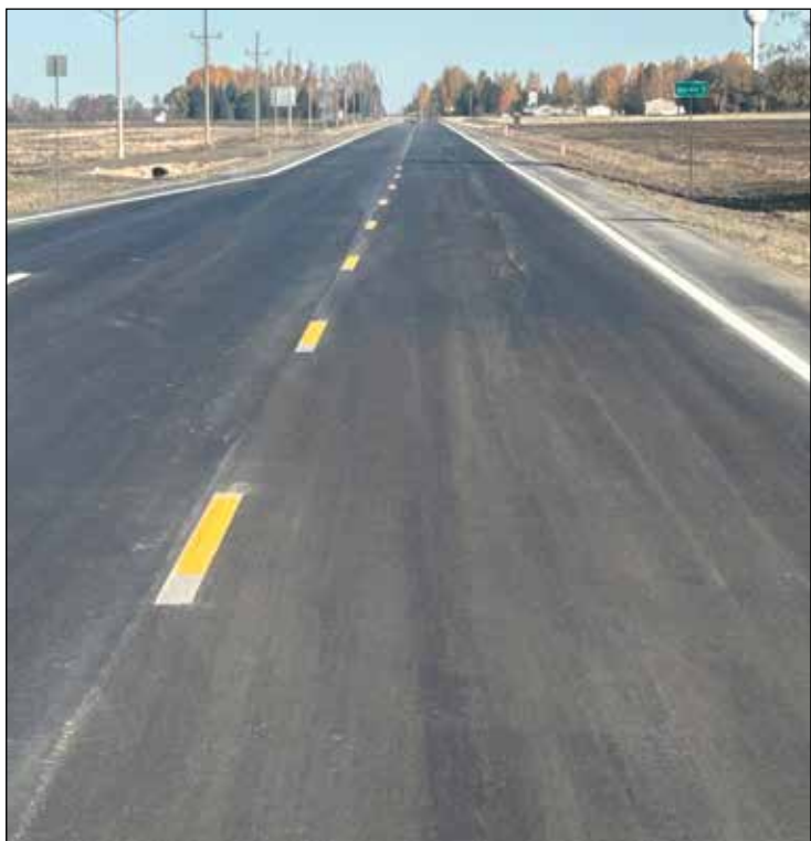
Striping is completed on the Oklee Construction Project.
