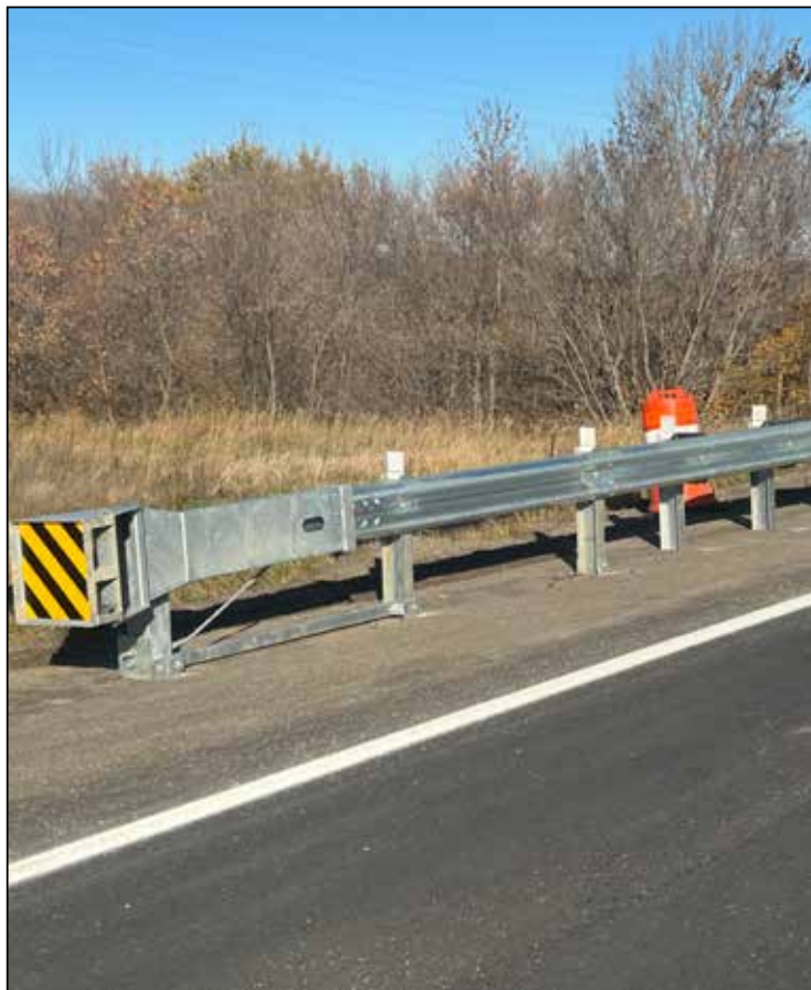
New Guard Rails on the bridge over the Lost River on the north edge of Oklee.
