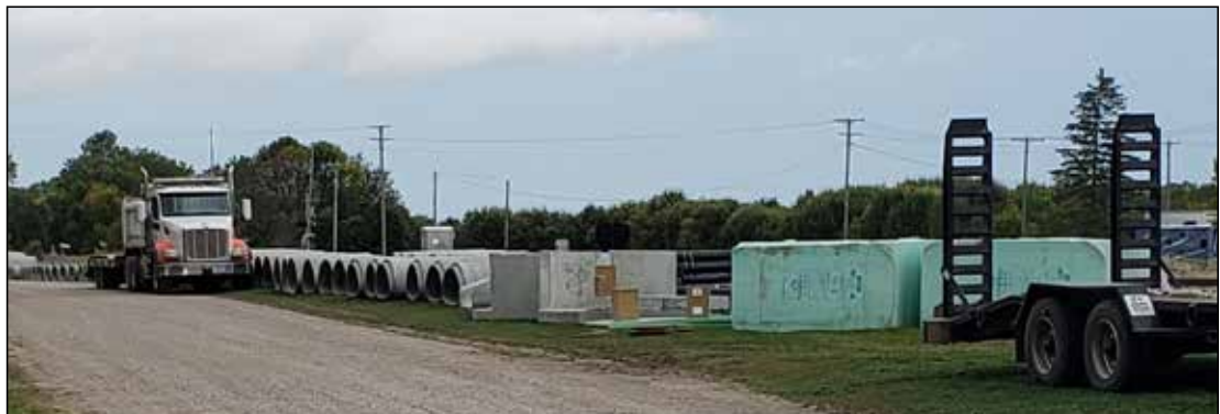
Lots of culverts and other supplies lying along the RR tracks in Oklee to be used in the reconstruction of State Hwy 222, now owned by county and renamed County Road 5.
