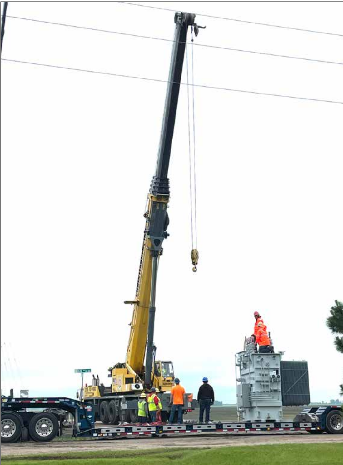
This large crane from Bemidji worked at the location of the new Otter Tail substation south of Oklee. Mary Lynn Bachand sent in the photo stating "I don't know that anyone else would be interested in seeing this, but it was pretty fascinating to watch this operation." Any changes in Oklee should be noted. Thanks for sending in.
