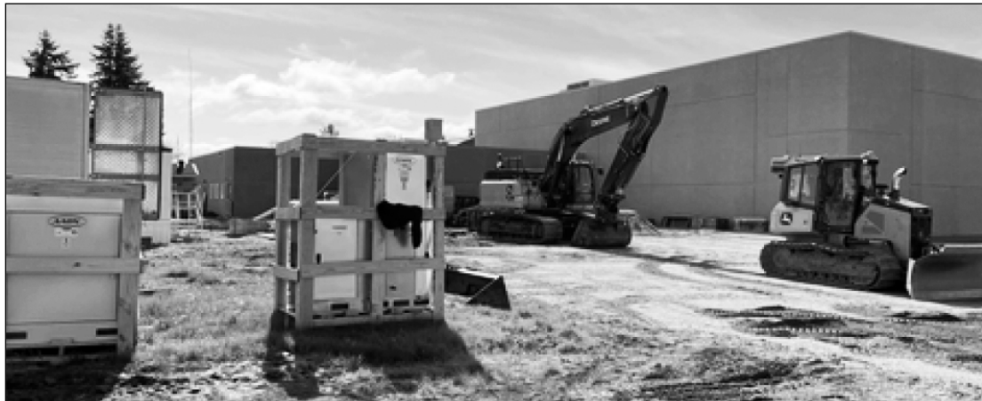
Parking Lot is being created next to the new gymnasium.
