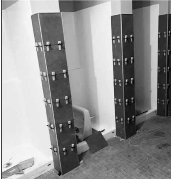
Tile worker installing tile in the bathroom and shower room.
