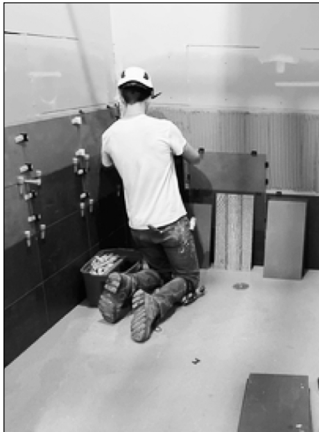
Tile worker installing tile in the bathroom and shower room.
