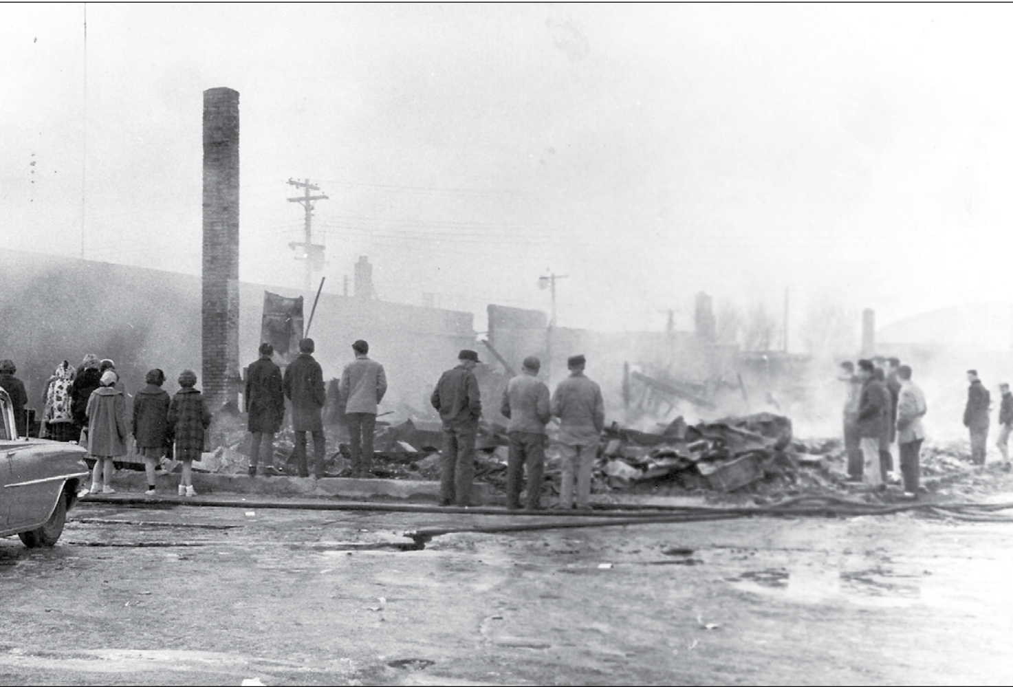
Only chimney remains standing of the bowling alley after $150,000 fire.
