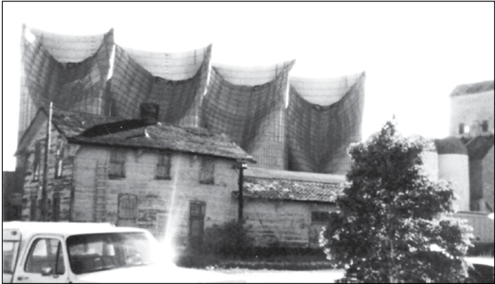
Oklee Farmer's Co-op Elevator bins damaged by the tornado that hit Oklee in 1982.
