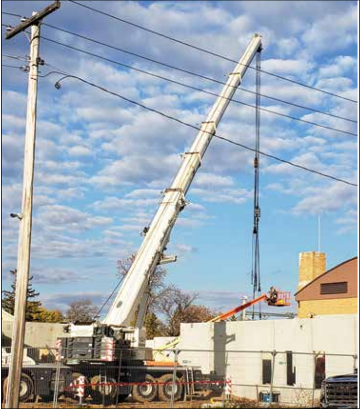
Work continues on placing the prefab walls of the new gym area at RLCC High School.
