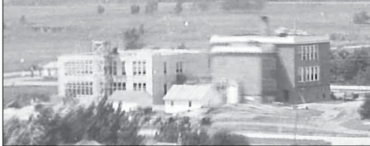
Picture of the 1939 building being built. Courtesy of the Oklee Historical Society.
