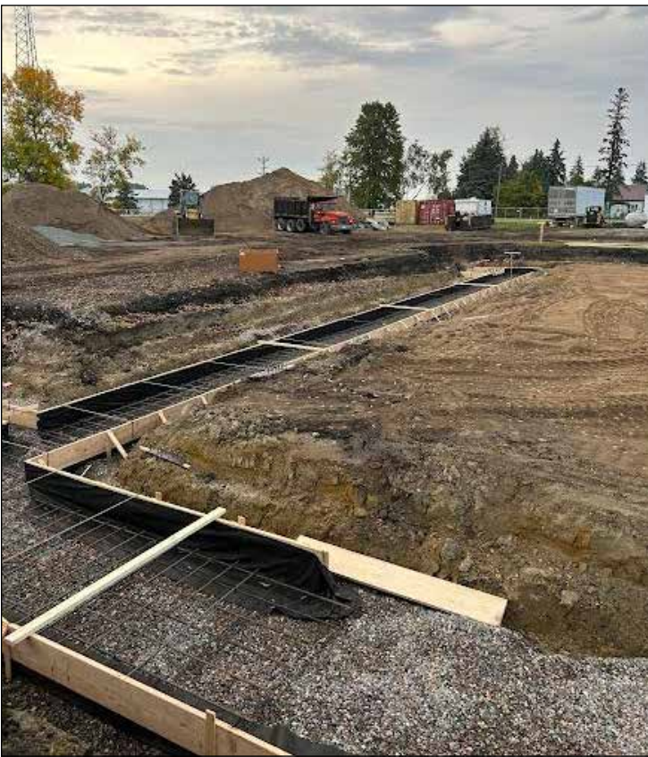
Current School Construction Photos by Eric Mickelson - The footings for the new gymnasium have been poured and reinforcement re-bar has been added.
