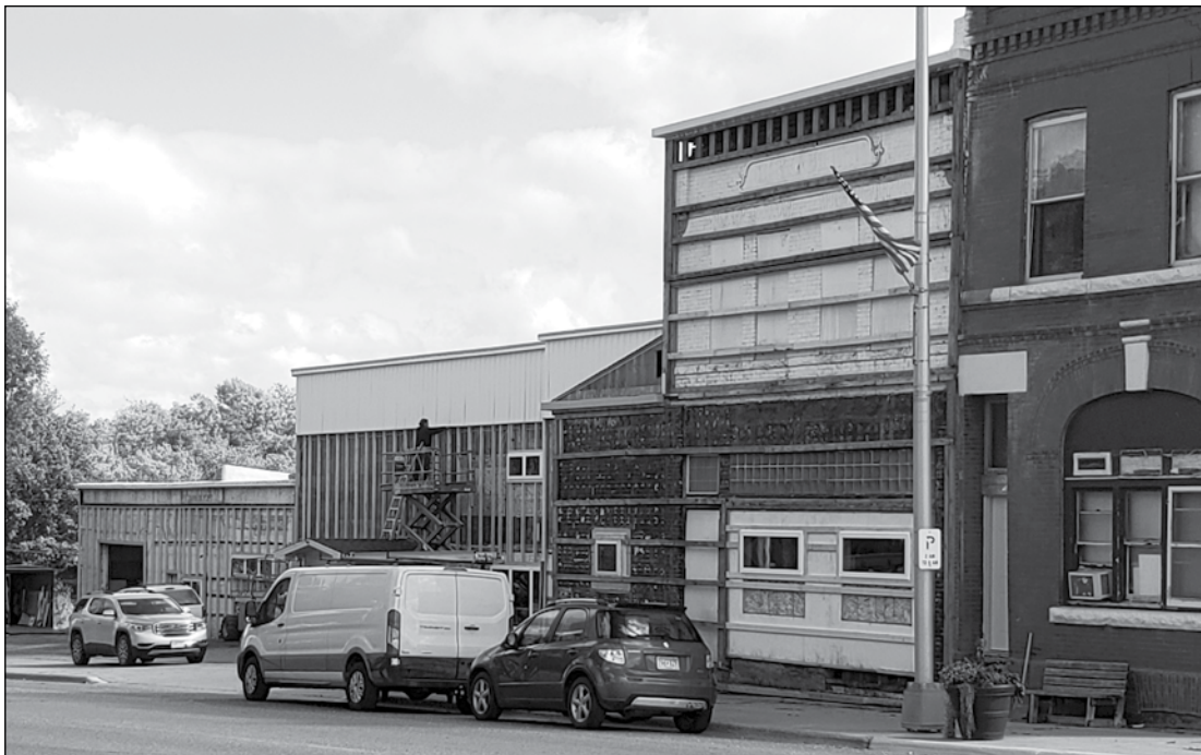
Wrights Consignment in Red Lake Falls is getting new windows and store fronts last week. That should help their heating bill. Looking forward to their new look.
