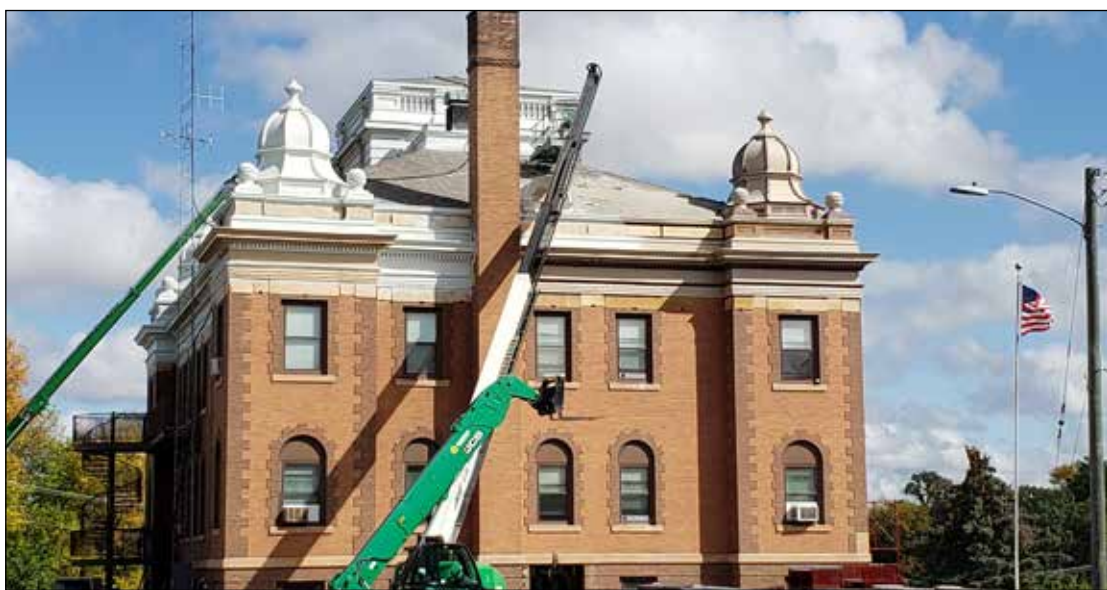
Work continues on the RLC Courthouse. They were busy painting the roof sections.
