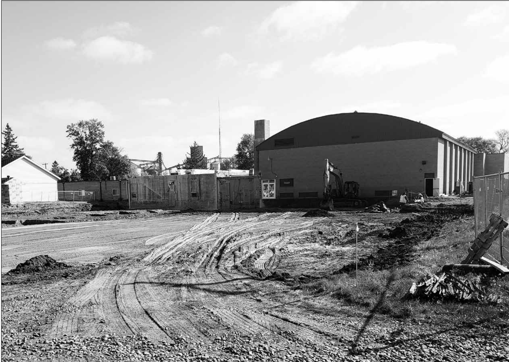
Ground work is being done to prepare for the new foundation of the new gym and other sections of RLCC High School.
