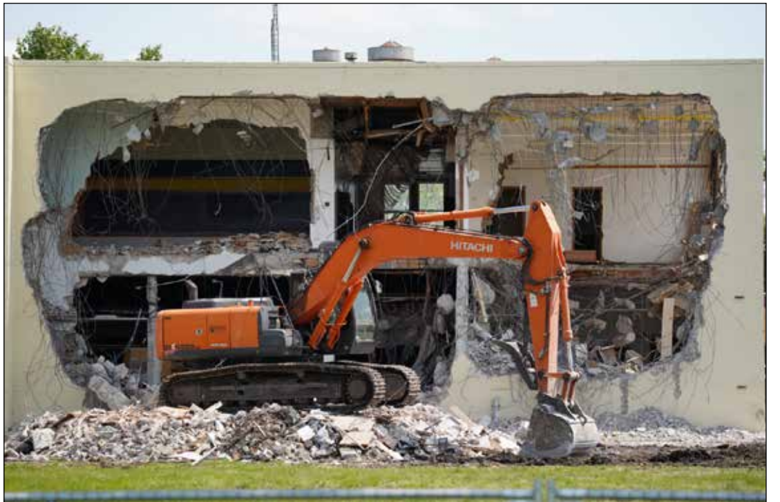
Pictured above: A backhoe is being used to pull apart the thick concrete walls in the 1939 building. Pictured below: The doorway to old classrooms will soon come down, almost to when one door closes, another opens.
