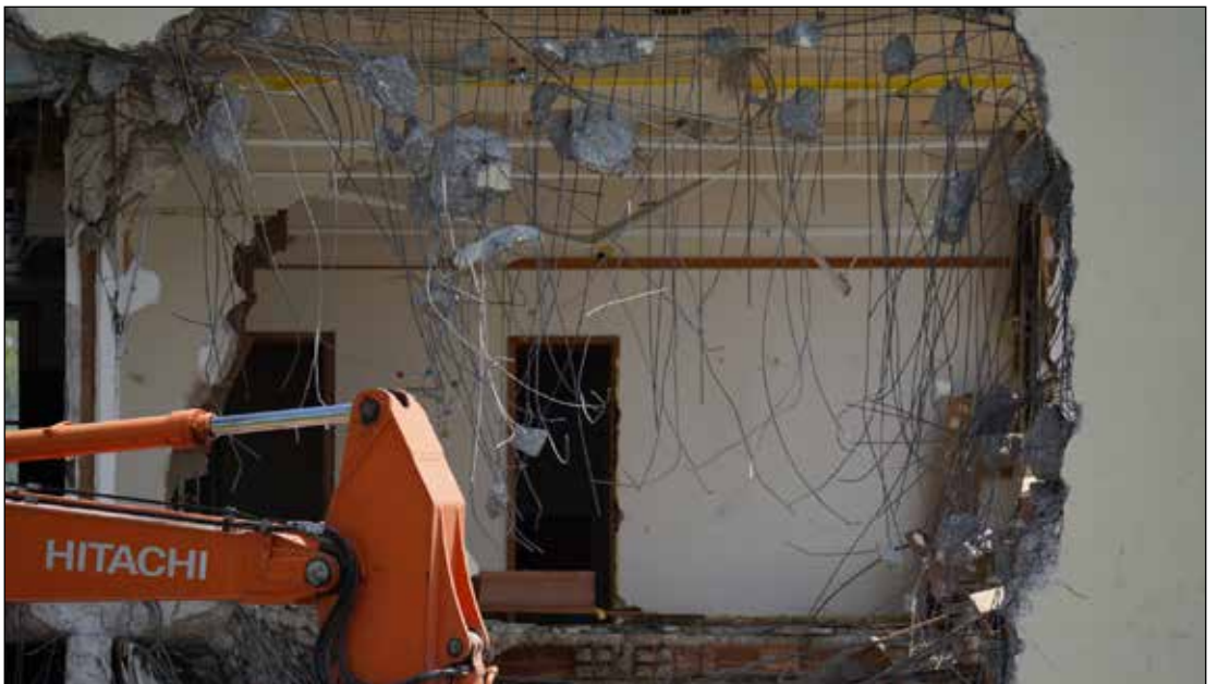
Pictured above: A backhoe is being used to pull apart the thick concrete walls in the 1939 building. Pictured below: The doorway to old classrooms will soon come down, almost to when one door closes, another opens.
