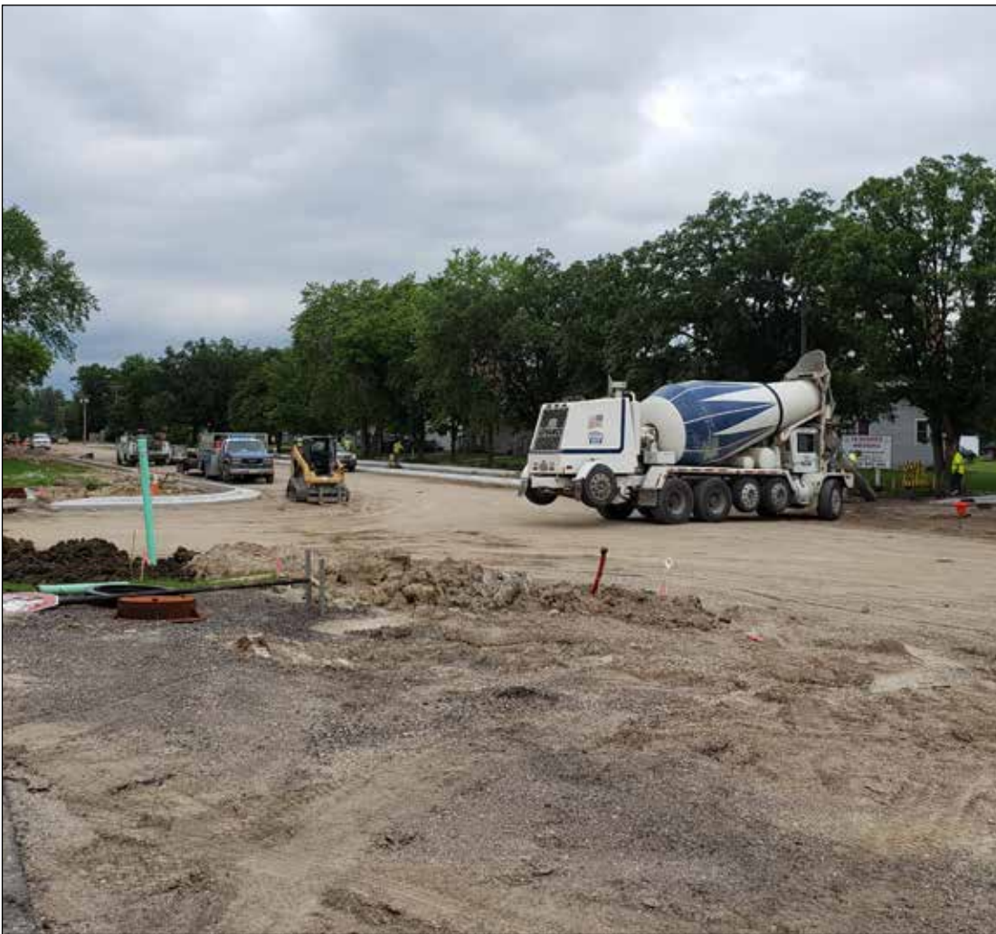
The western end of Plummer was getting curb and gutter work completed as the rest of the crew moved eastward for more sewer, water and waste pipe work was completed. Many piles of sand and gravel dot the area.
