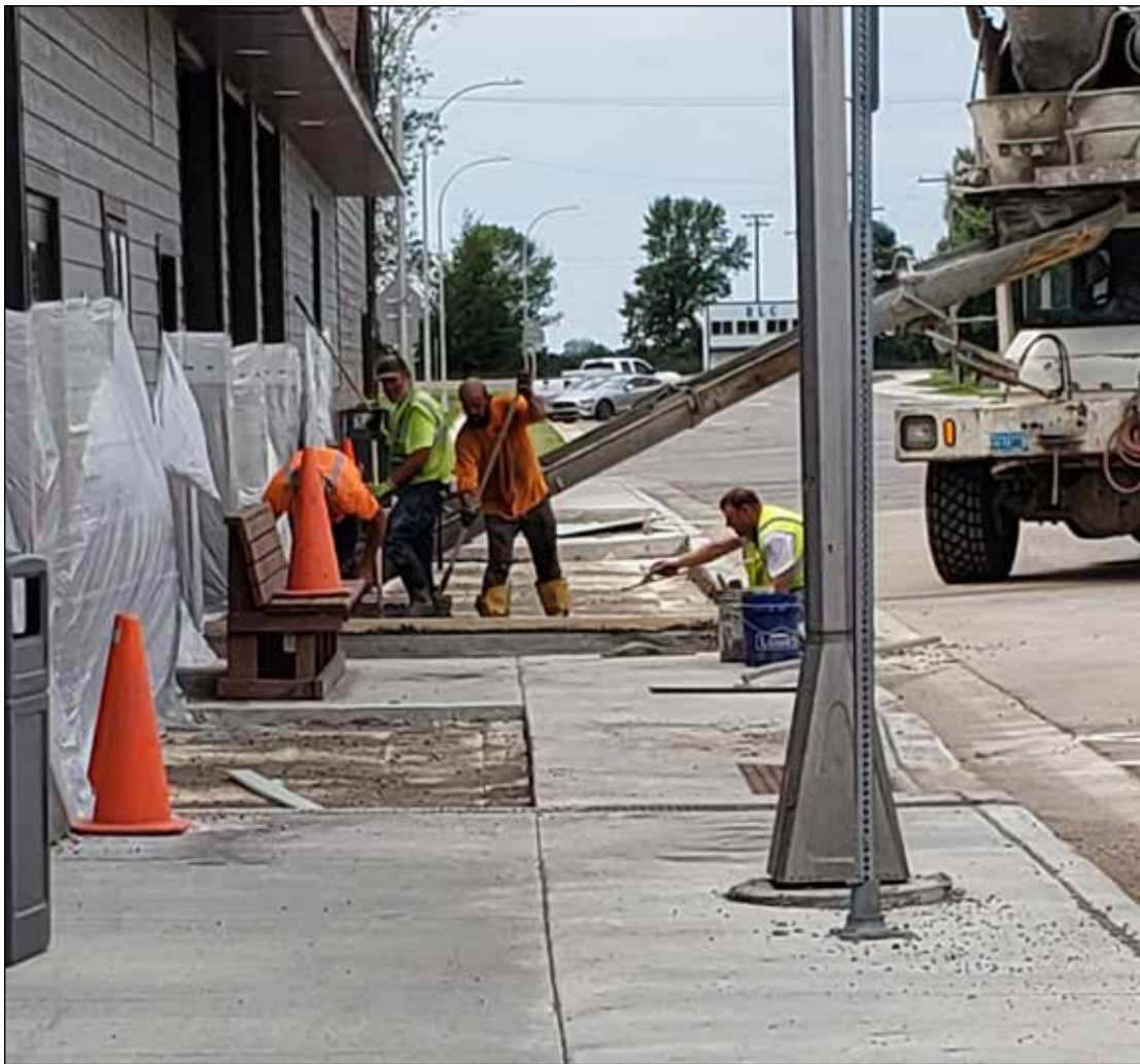
After some winter trouble with sidewalks raising in front of some business doors after the construction last year on the County Roads in Oklee, they were chopped out and new concrete was poured a couple of days last week.
