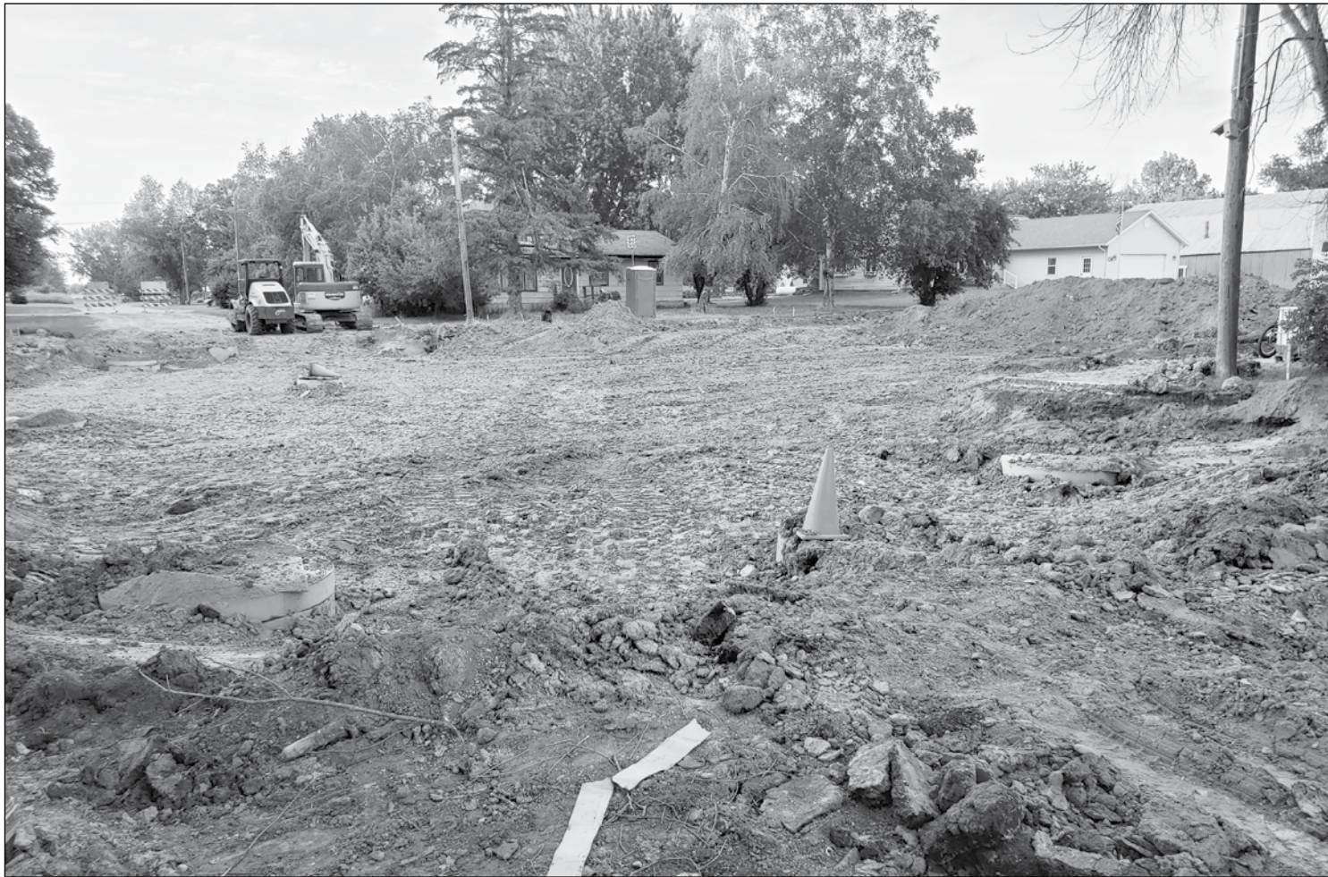
The street work in Plummer is progressing, unfortunately it makes it hard to get around town easily. As you can see in this photo of Main Ave, one block west of Minnesota Street, there is lots of work left to do before it is open for traffic. New concrete storm drainpipes and sewer and water lines have been place.
