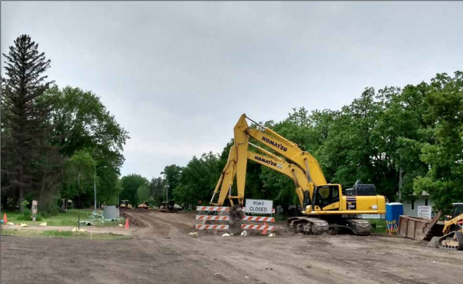
Two excavators in front of the County Shed on Central Avenue looking west.
