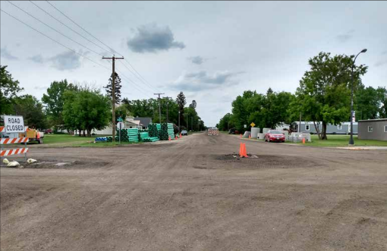
Stacks of Water (blue) and Sewer (green) pipes on the side of the road have not been installed yet. This is the corner of Minnesota St and Center Ave, looking north.
