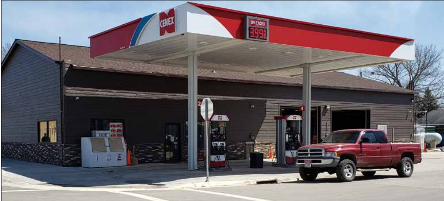
Cenex C-Store in Oklee got new shingles and siding. They matched the strip piece on the City building and complemented their building with stone. It looks very nice.
