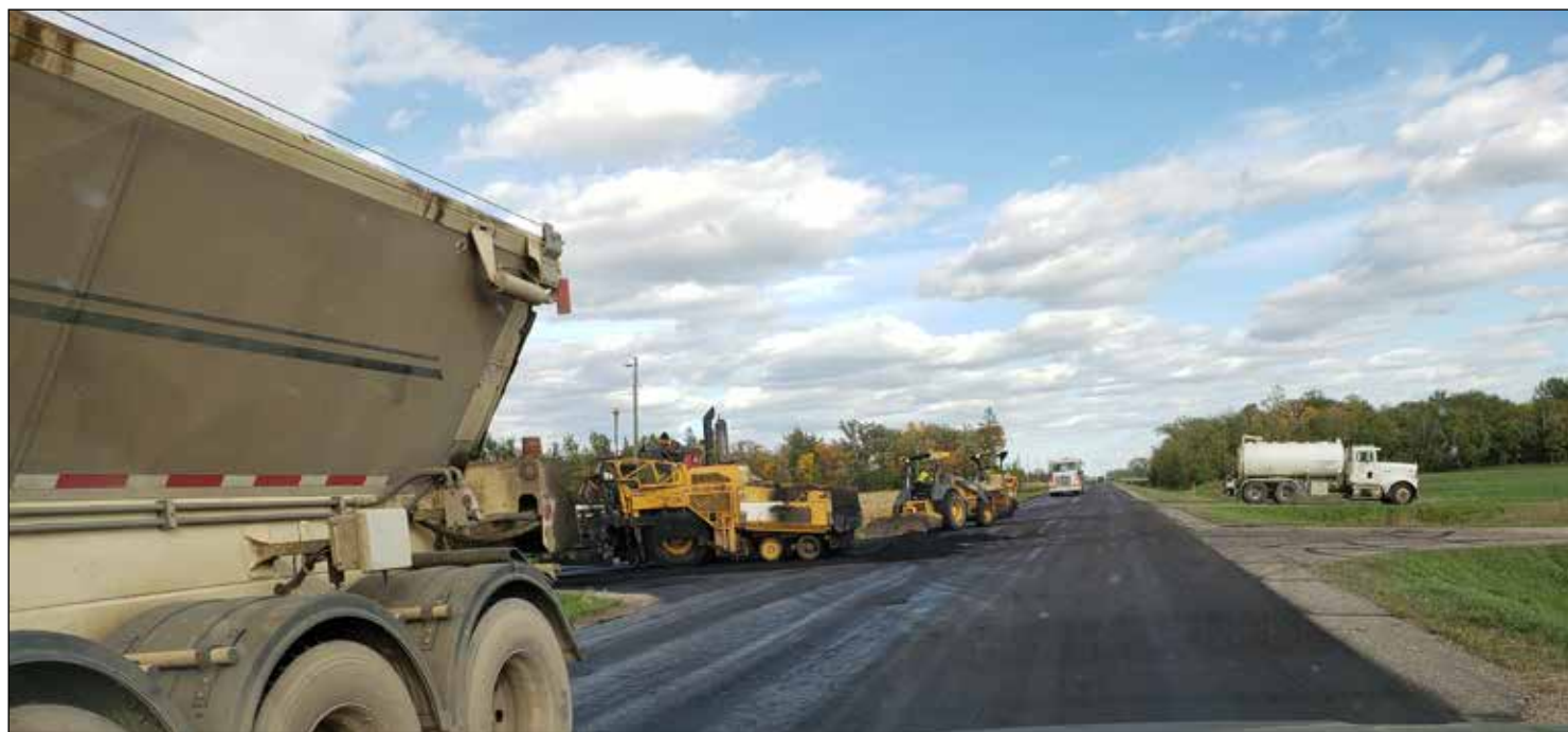
Road work continues on Red Lake County CSAH #6 east of Oklee. Be careful, it is also harvest season in the area.
