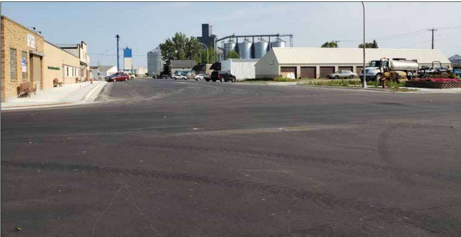
The tarring of the county roads through Oklee are completed, though there is some small pieces of the project to still be done, but the major portion is done and people can now walk and drive downtown without issue.
