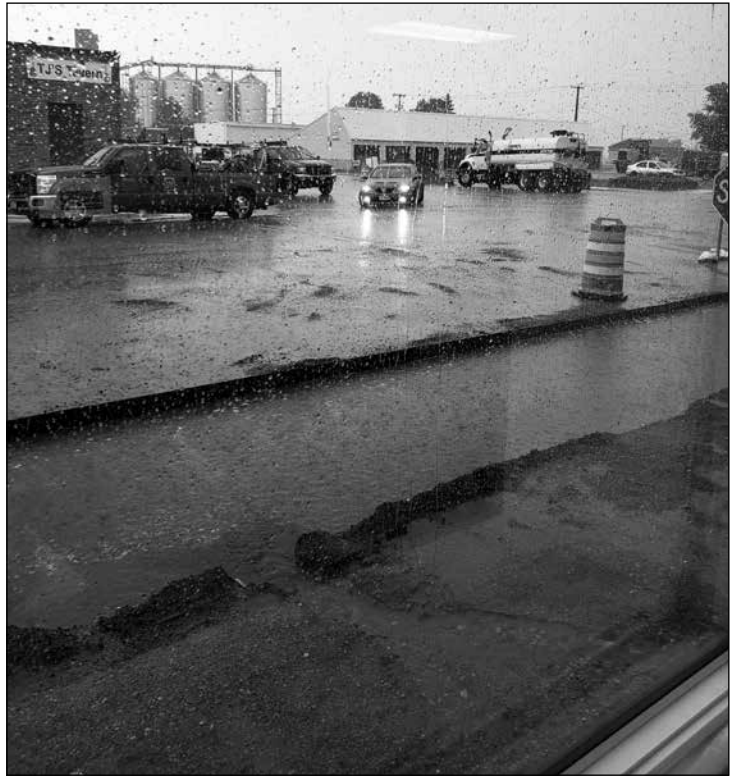
Picture from the window in the Oklee Herald office on Monday around noon. Rain pouring down and filling the areas where the curb and gutters are going to be.
