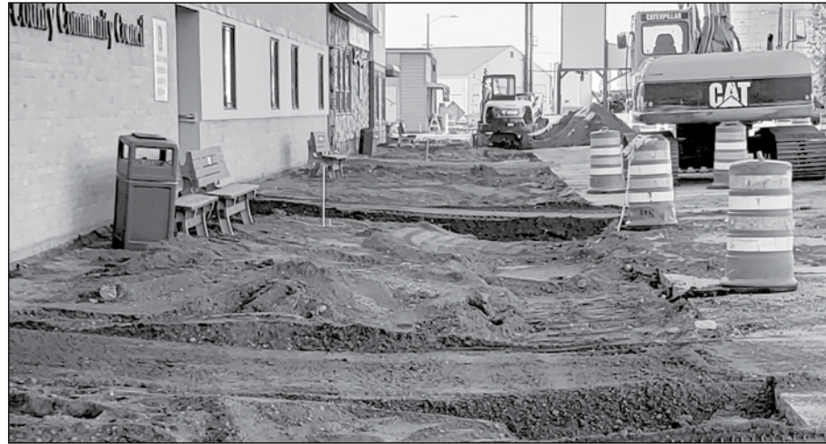
1st Avenue looking west - and looking east. The old curb and gutter has been removed and they are ready to start putting forms down for the new sidewalks and gutters. Below: the entrance to the bank and Main Street have temporary paths in place.
