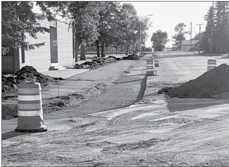
1st Avenue looking west - and looking east. The old curb and gutter has been removed and they are ready to start putting forms down for the new sidewalks and gutters. Below: the entrance to the bank and Main Street have temporary paths in place.
