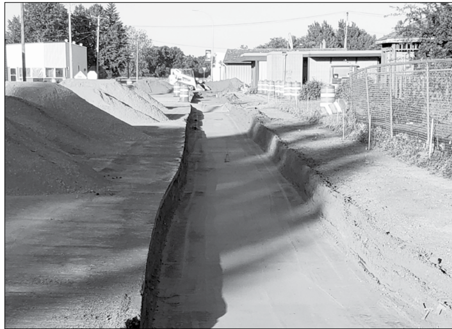
1st Avenue looking west - and looking east. The old curb and gutter has been removed and they are ready to start putting forms down for the new sidewalks and gutters. Below: the entrance to the bank and Main Street have temporary paths in place.
