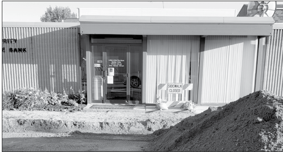
1st Avenue looking west - and looking east. The old curb and gutter has been removed and they are ready to start putting forms down for the new sidewalks and gutters. Below: the entrance to the bank and Main Street have temporary paths in place.
