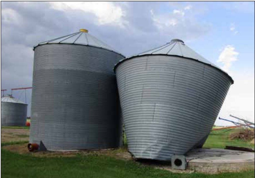
O'Neill's lost one grain bin. The wind must of been straight line winds to pickup the machine shed roof and push over the empty grain bin.
