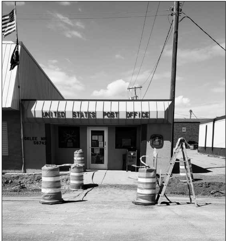
This week, the front of the post office will not be open. You will have to go to the back door to pick up your mail as the curb and gutter are being put in.
