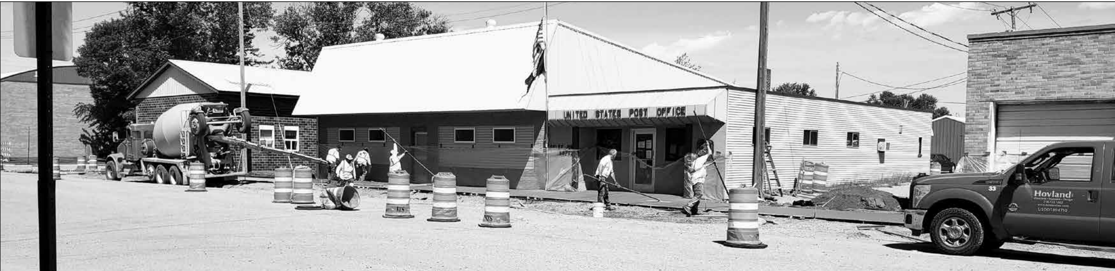
Part of the sidewalks from the RLCC School corner to TJ Tavern were being poured and screed on Monday Morning. Post office access is definitely from the back door this week.
