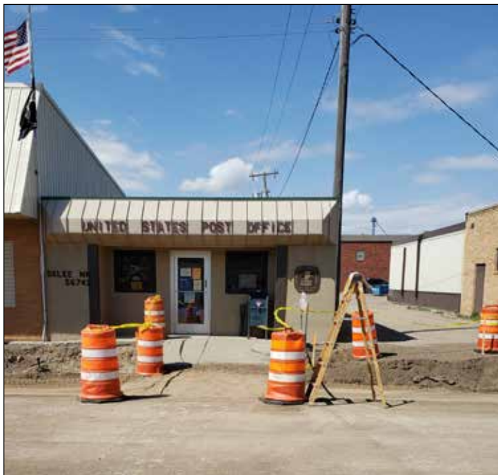
As the work continued west down 2nd Ave on Wednesday and Thursday last week, you had to come in through the alley to access the post office. On Friday, they put in a temporary entrance until it is time to put in the concrete for the curb and gutter.
