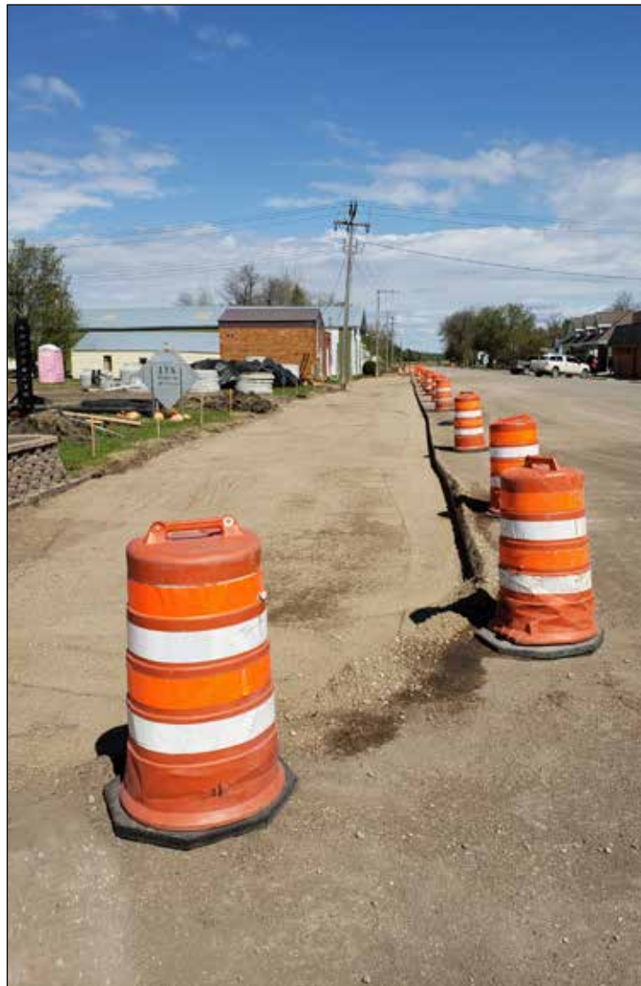
Looking east from Main Street down 2nd Ave. the dirt work is completed and ready for the concrete work. Crews still have more places to remove the old curb and gutters. Be careful where you park and walk while this project is being done.
