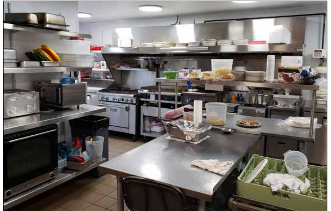
Kitchen was expanded and a CharBroiler and new 6 burner stove with oven were added. The cooler was expanded and a new walk in freezer was built.
