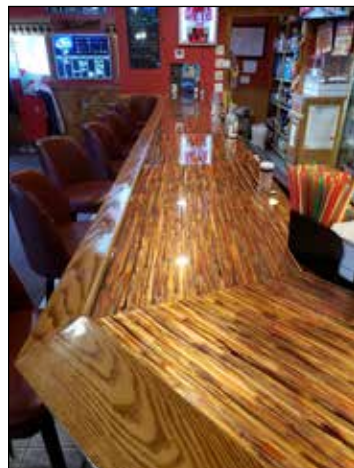
Beautiful new top was installed, etched copper and sealed with polyurethane.
