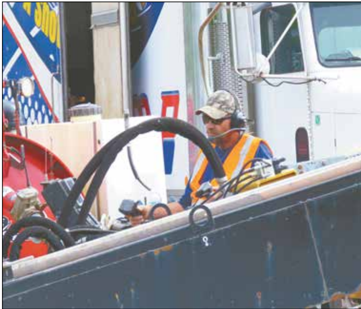
Guiding the lines going underground.
