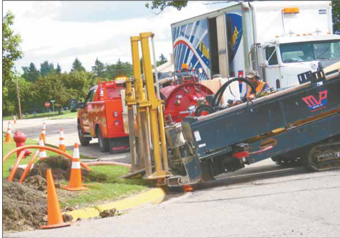
Takes lots of equipment to get in the underground lines.
