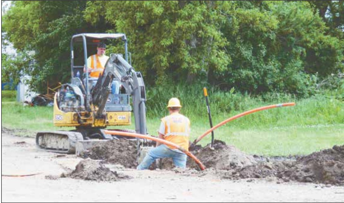
Company at work putting fiber optics underground.
