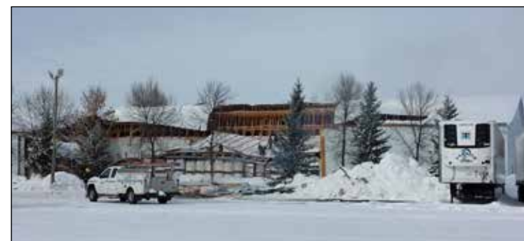
Last year in February, Paradis Storage building had part of its roof collapse.
