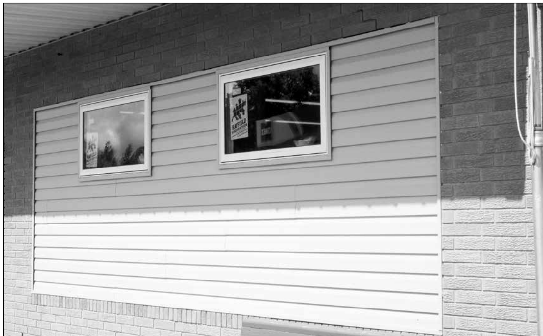
The new windows in the RLCC Shop building have been installed.
