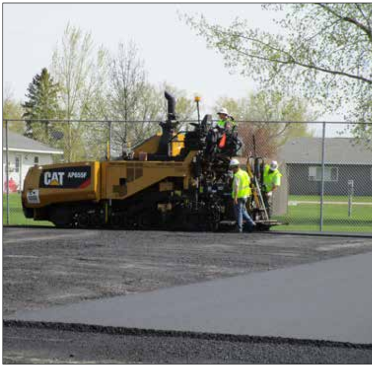
May 14th, the old tennis courts in Oklee got a new surface laid down.
