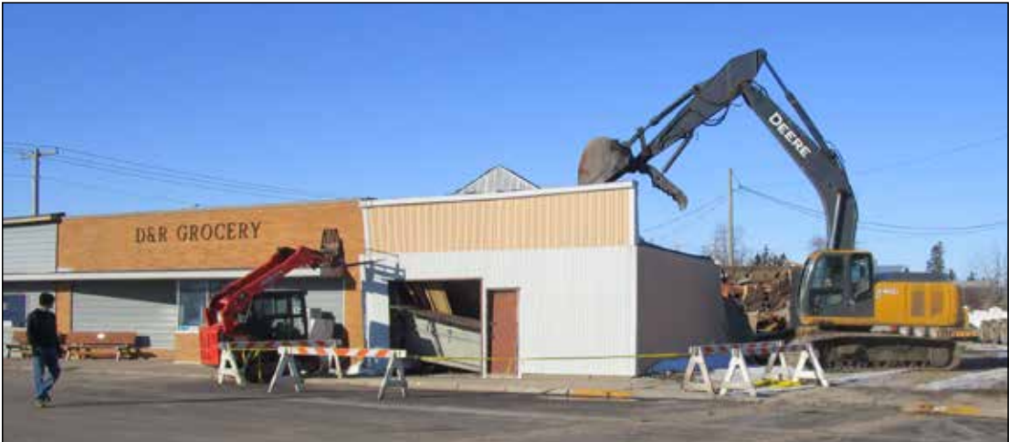
On Friday, Ryan's Backhoe tore down the old building to the north of D & R Grocery, which they used for storage.
