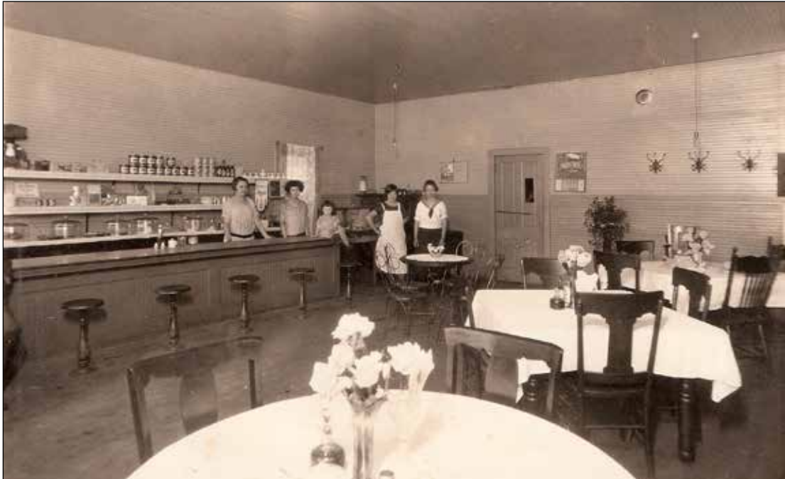
Early photo of the building Oklee lost this winter (D & R Grocery storage building). It has served as a restaurant and many other business over the years.
