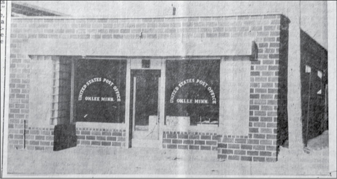
New Oklee Post Office: Patrons of the Oklee Post Office were serviced for the first time this morning (January 21, 1960) from its new location in the former Oklee Cleaners building. All equipment is new, including the 250 lock boxes and all furniture and equipment. The office was moved Wednesday from the Falardeau building on Main Street where it has been located since 1942.
