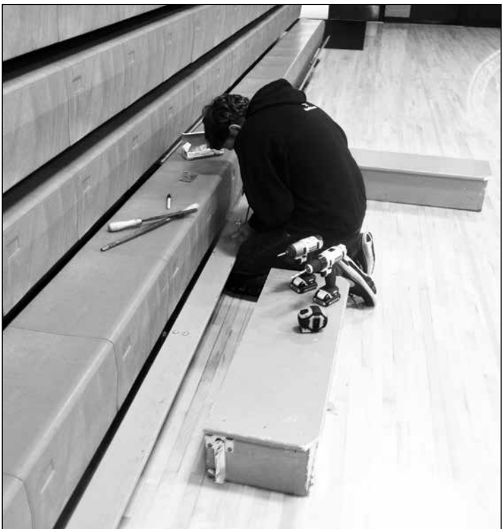
Tyler Jensen's project for his Special Projects Class is fixing the steps for the bleachers.
