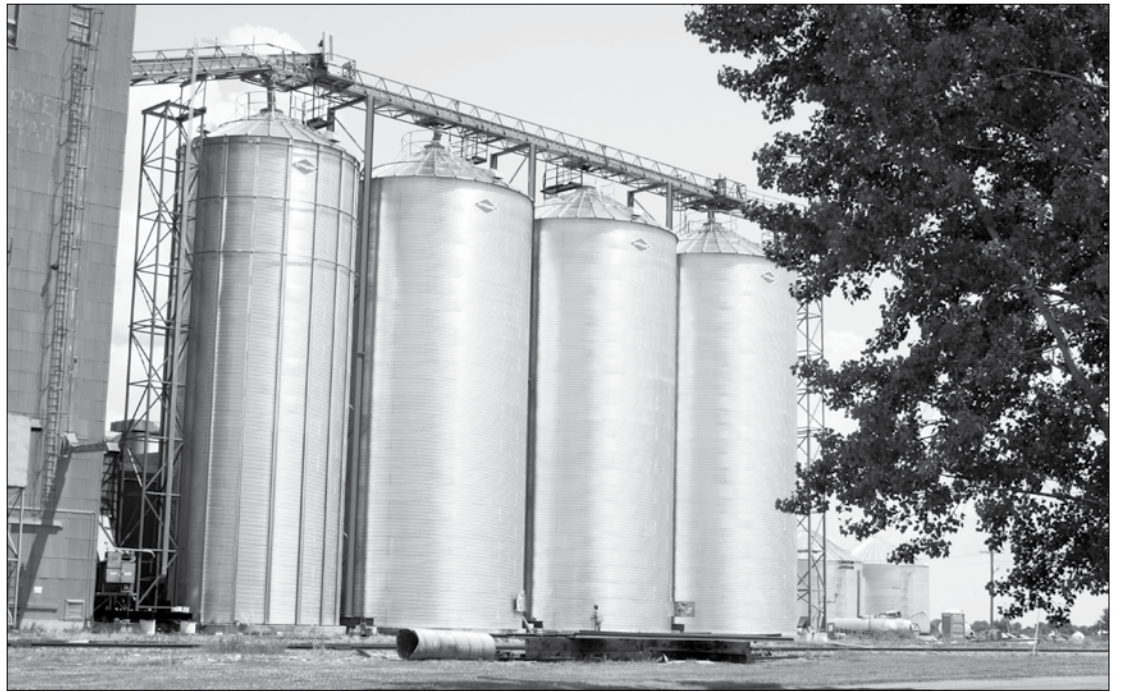
Northwest Grain/CHS, this spring, removed four of their bins and now the replacement bins are now in place for the fall harvest which will begin soon.
