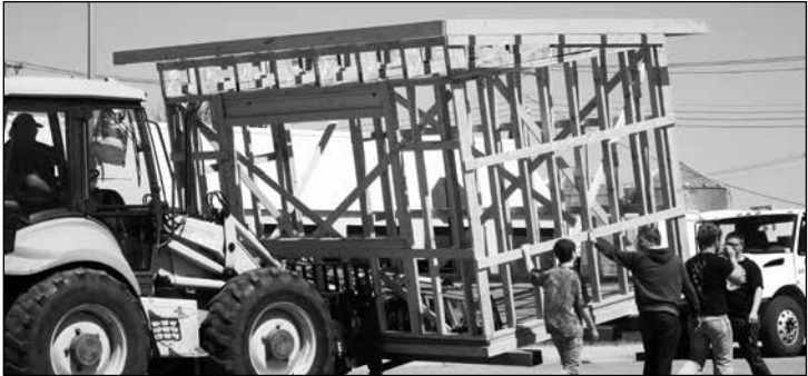
The RLCC Shop Class teacher moving the new concession stand to the baseball fields to be finished with siding and a roof.
