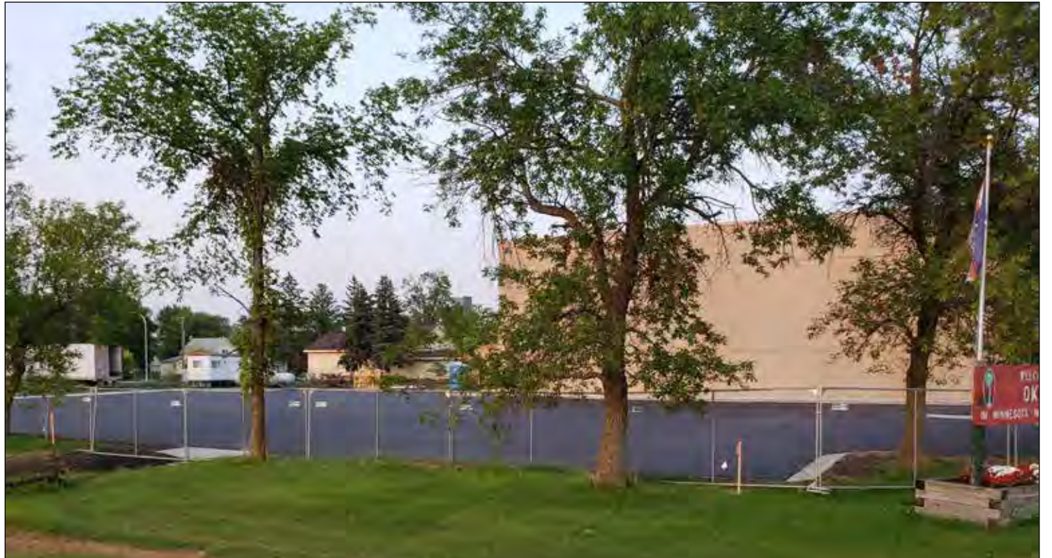
If you have been in Oklee recently and drove by the RLCC High School, the outside of the building is starting to look good. The roads and curbs have been tarred and replaced and the new parking lot for staff has been completed. Just a little landscaping left to do.
