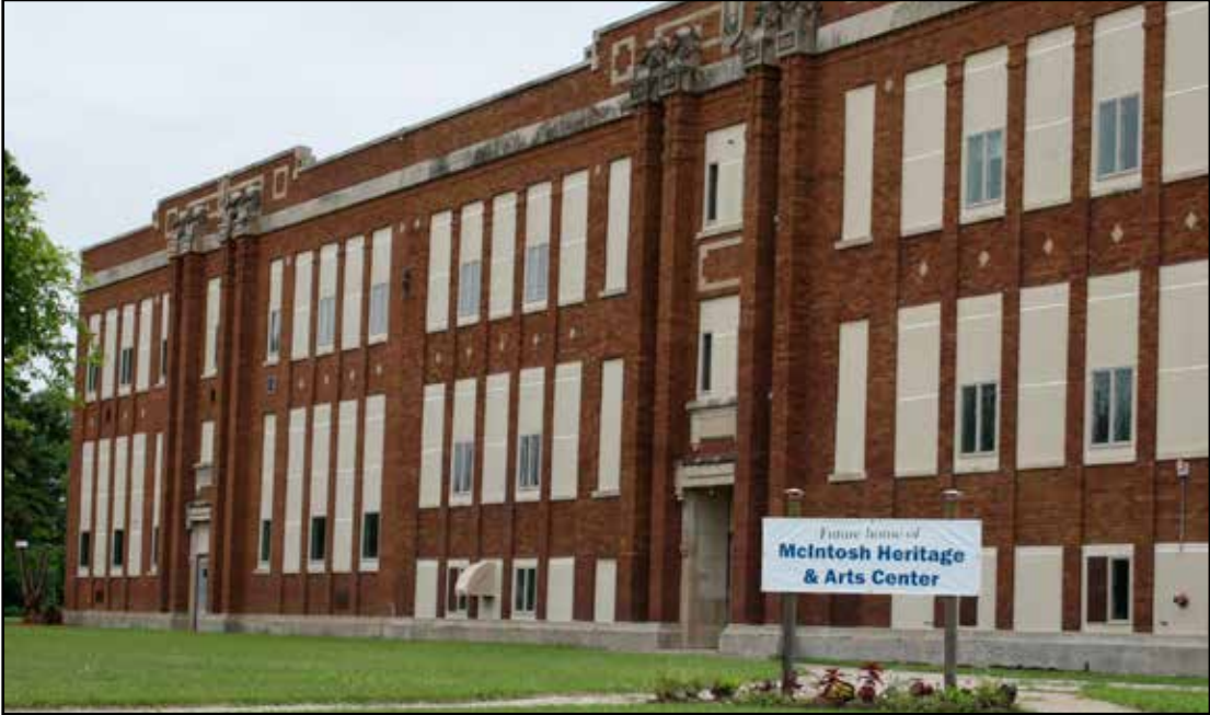
The old McIntosh School now boasts a new sign stating that is is the “Future home of McIntosh Heritage and Arts Center” along with a beautiful flower garden to rest in. MHAC continues to raise funds for the renovation of the school. The yard has been a focus this summer with new art, tree trimming and flower gardens.
