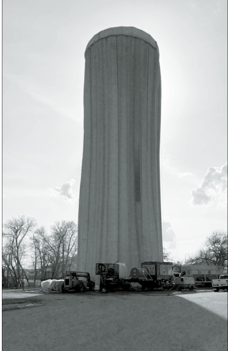
Casting a large shadow, the McIntosh water tower is fully curtained to control the spray from sand blasting.
