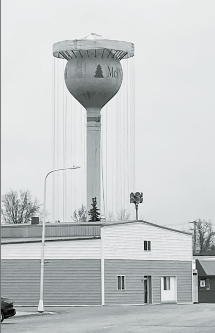
The crew working on the McIntosh water tower prepare to curtain during sandblasting.
