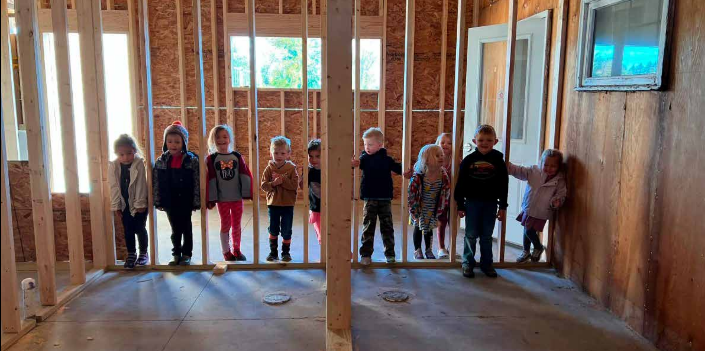
The Clubhouse Childcare Center preschoolers had fun checking out their new classroom. The Clubhouse, located in McIntosh is happy to share that they are adding on a new preschool suite. A fun fact: there are 4 Clubhouse dads and 2 Clubhouse grandpas contracting and working on this project!
