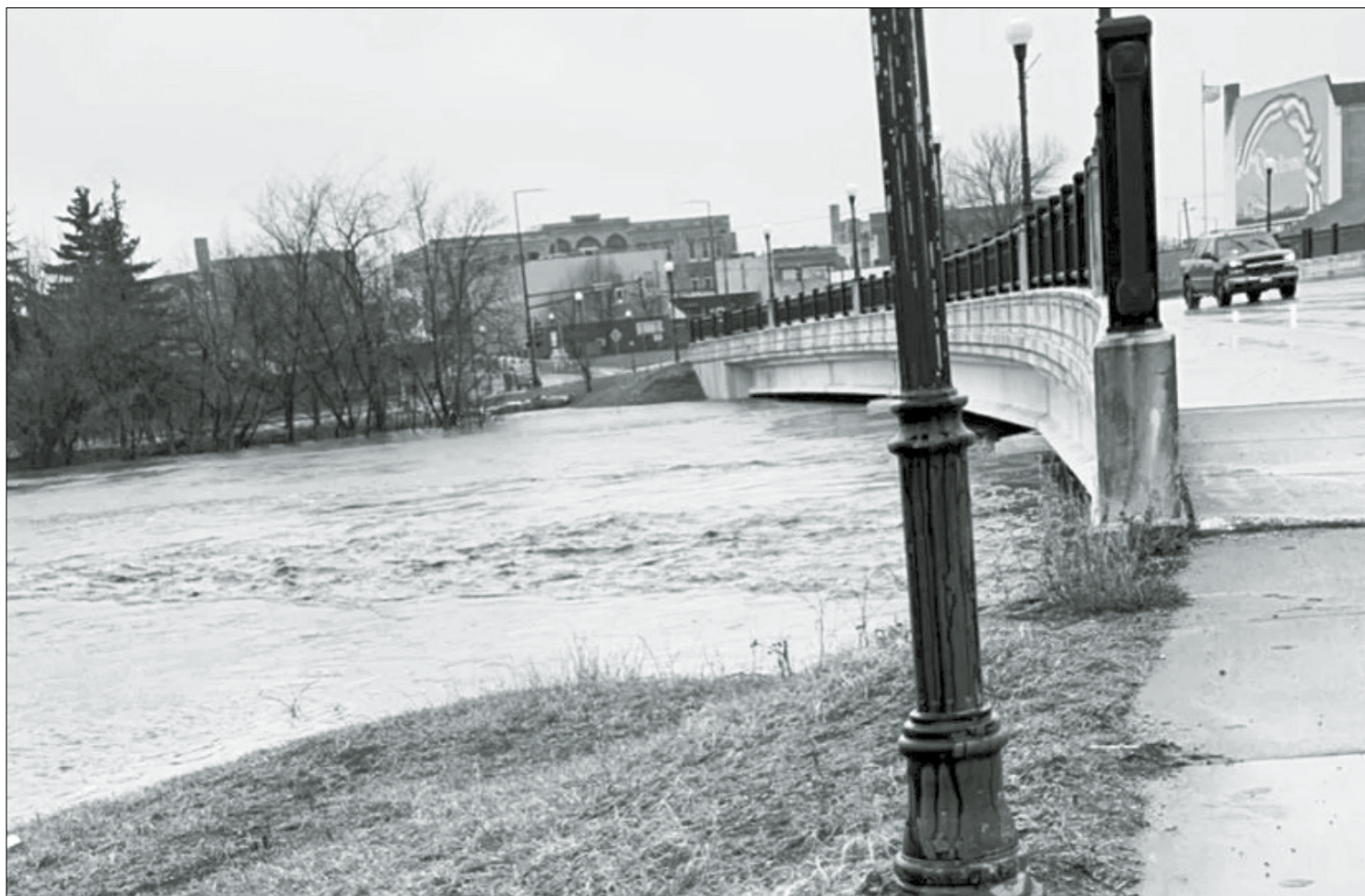
The Red Lake River flowing through Crookston reached the height of the bridge on Saturday afternoon. Crookston is currently in a State of Emergency due to flooding.
