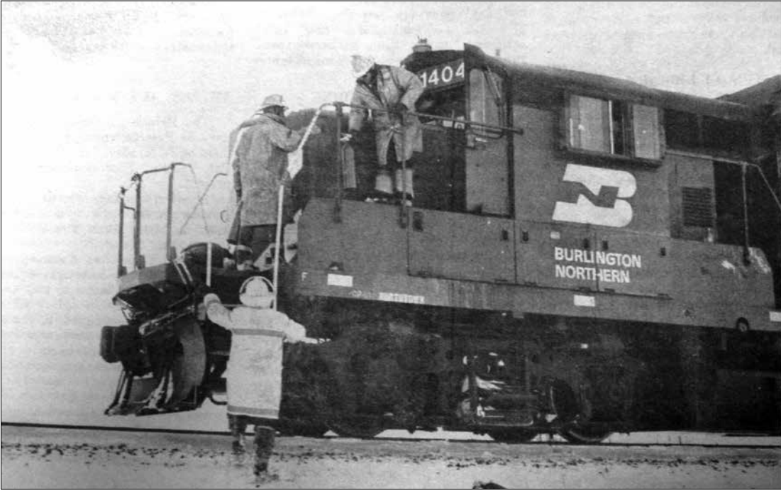
40 years ago...1982: At about 3:45 pm on Monday afternoon, Burlington Northern's Locomotive Engine No. 1404 called in an alarm to the McIntosh Fire Department. The train was on the tracks about a mile west of McIntosh. The engineers first noticed the danger when it began to get smoky in the cab. The problem was apparently an electrical fire in the generator. The engineers reportedly saw three foot flames shooting from the generator when they opened the door. The flames subsided before the firemen arrived but shot up again and the firemen were able to extinguish them with the portable chemicals. Boarding the locomotive were McIntosh volunteer firemen: Tom Bauer, Craig Burslie, Russ Horacek, John Middleton and Jim Wertish. Also responding to the call were Melford Grundyson, Richard Keller, Clyde Kringlen, Dick Parent, Sherman Tranby and Jerry Wertish.
