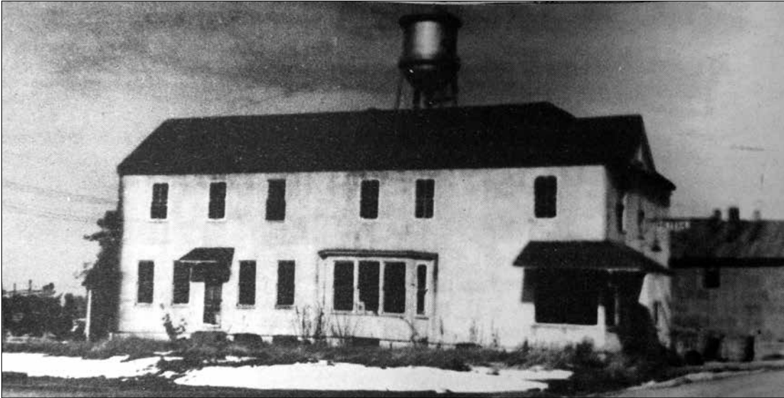
50 years ago...1970: Make way, traffic coming! This dilapidated building above would hardly be recognized as the social whirl of McIntosh, but it had its day! It is the hotel building which will be razed to make way for the new construction on Highway 2. It has undergone many changes and several remodels under many owners. Obviously its usefulness is over. The hotel was once the center of business and social activity of a bustling McIntosh in the 1910 era. Though at one time there were three hotels in McIntosh, this was the largest and most ornate. It dominated the village scene earlier than 1894, as a stopping place for traveling salesmen, immigrants and tradesmen. Ole Johnson built the first hotel in McIntosh, a man by the name of LaBree built the hotel in its present location in 1889. It was later sold to Ed West who built an addition to it, and it went by the name of West Hotel. After West, Hans Bolstad bought the property and Michael O'Brien purchased it about 1909 and owned it for about 18 years. In recent years it has belonged to Levor Bjella who has rented it out to a number of operators.
