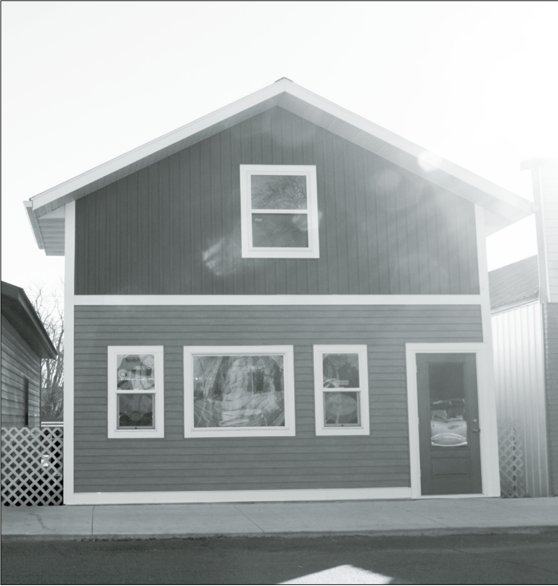
Along with a new sidewalk this summer, Kingtown Mutual Insurance Company recently had new siding put on their building on Cleveland Avenue in downtown McIntosh. The new siding gave the building a fresh and updated look.
