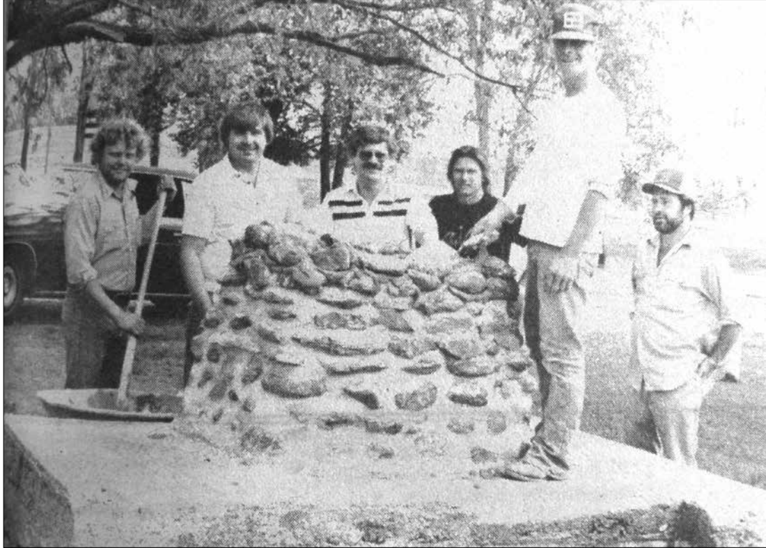
40 years ago...1980: Dean Strom is the foreman of the Men's Action Crew (Mac's) rebuilding the park fireplace in the Roholt City Park. This is a volunteer project by our community men.
