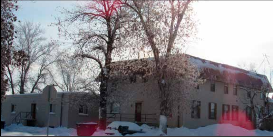
A fire in the lower level of the See-Bee apartments caused residents to be evacuated early on Monday, January 17th. There was damage in a single apartment, and residents were able to return to their homes later in the week. The cause of the fire was an oven left on during a resident's absence.
