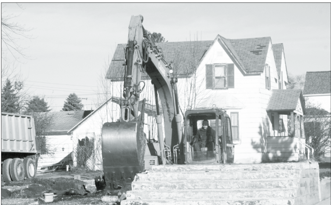
The steps of Salem Church are all that remain of the Church. The final phase of the demolition took place on Monday, November 9, 2015 as the foundation and steps were removed and the area was filled.
