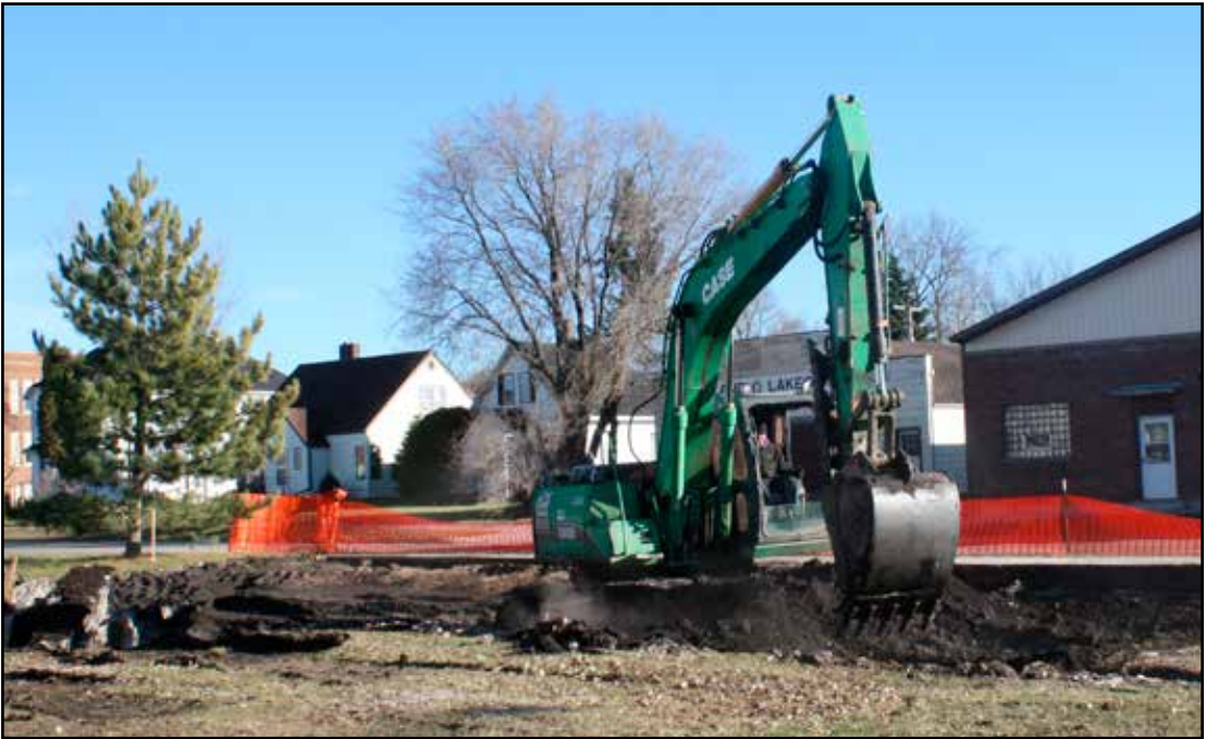
Saying goodbye to Salem: The final work was being completed on the removal of Salem Church on Monday, November 9th when the foundation and stairways were being removed and the hole was filled.
