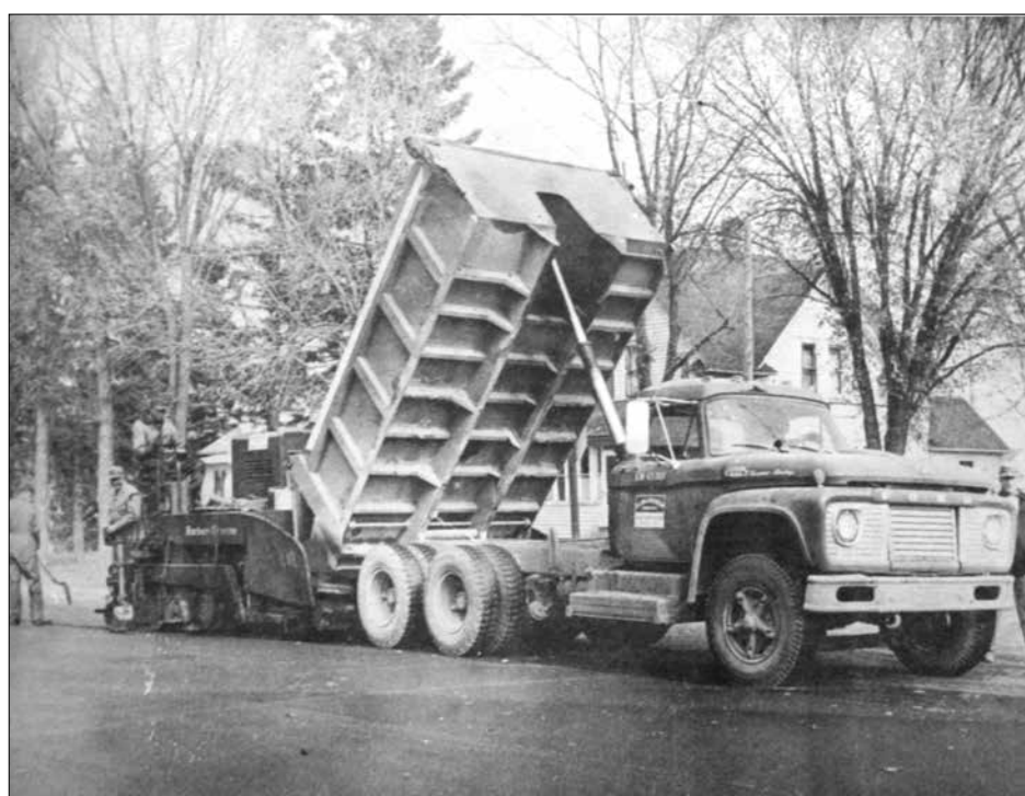
50 years ago...1969: Street surfacing nears completion in McIntosh as crews of the McLaughlin company took advantage of the warm, sunny days over the weekend to lay the two inch asphalt carpet.
