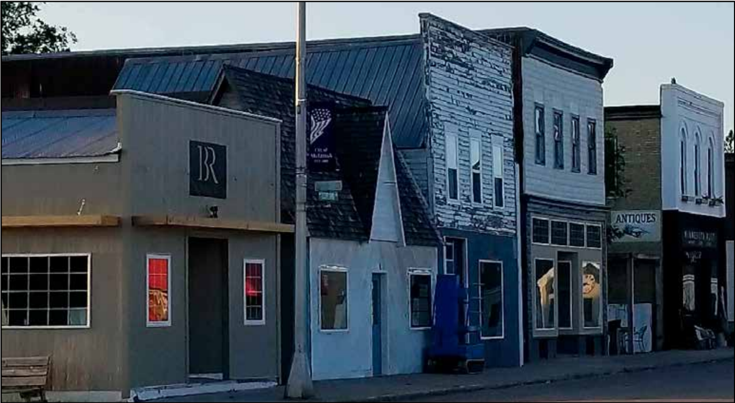
Recent renovations to downtown McIntosh as 4 buildings on the west side of the street receive updates and make space for some new business. Stordahl Construction is doing the renovating.
