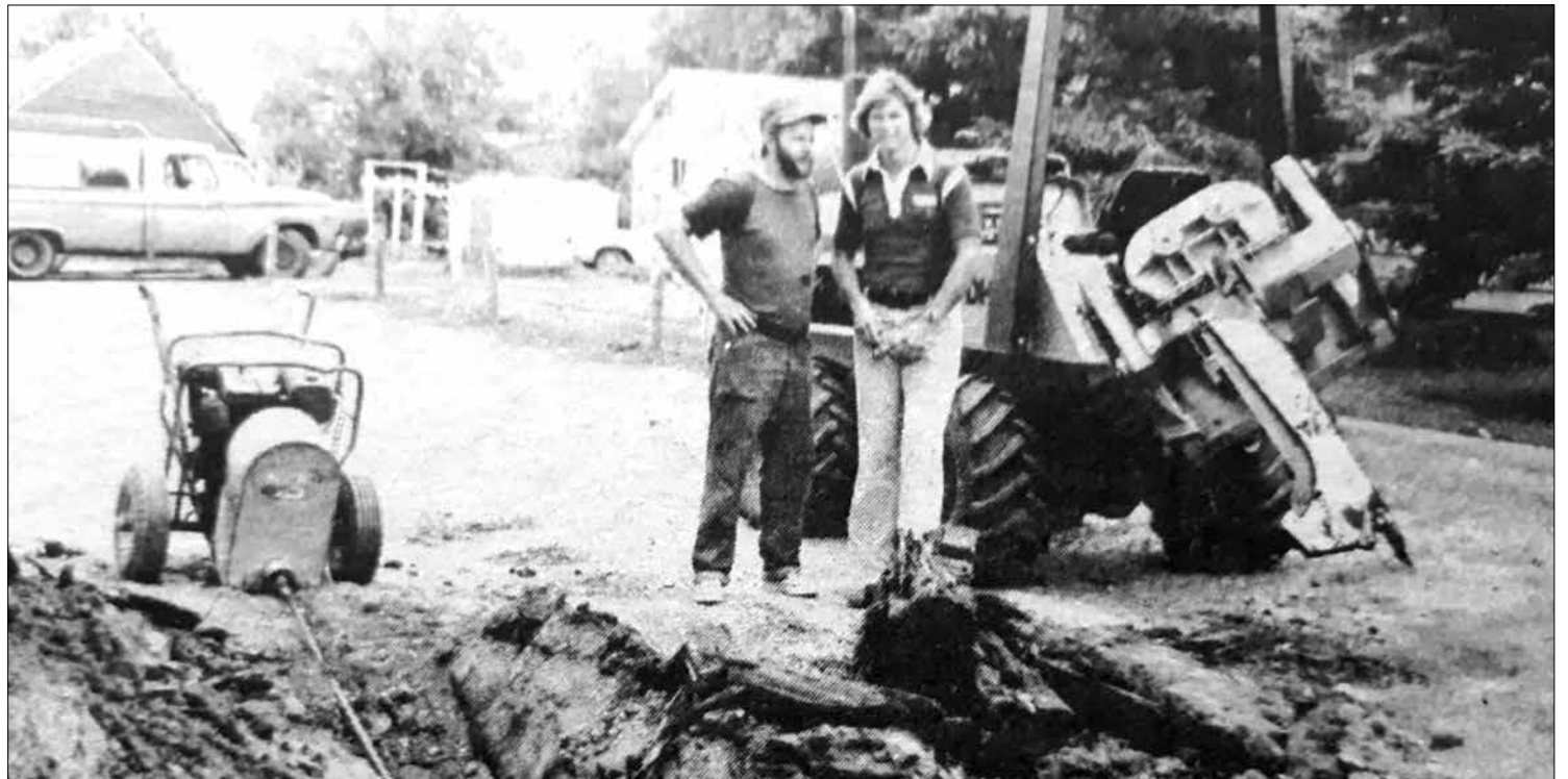
40 years ago...1979: Cable TV is coming into McIntosh. Rocky Schlichter with Cable System Services working with 3-M Company putting in cable TV and telephone co-axel wire with the use of this small equipment used in the city and is standing with Bruce Haaven with Garden Valley Equipment. Hook-up for cable TV should take place in the area by late Fall.
