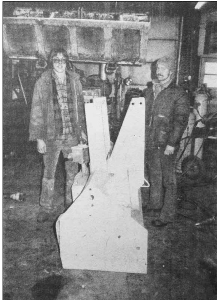
40 years ago...Two young men from McIntosh who work at the Erskine Manufacturing Inc. are Todd Tranby and Cal Schow. Todd is assembling a gear box into the blower and Cal runs the cutting torch and makes parts in the manufacturing section.
