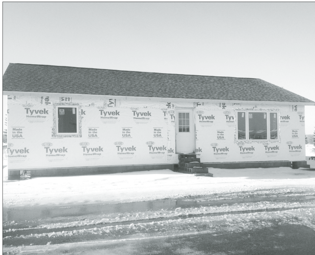
The Construction Trades students at Win-E-Mac School are constructing a house that will be moved to a permanent location and is for sale.
