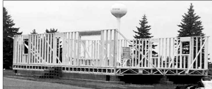
The Win-E-Mac Construction class has been working hard on building a new house. If you would like to view their progress, it is located in back of the school.
